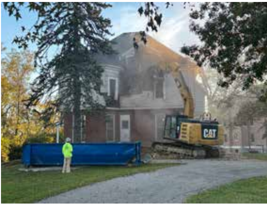
Demolition of St. Joseph House.
